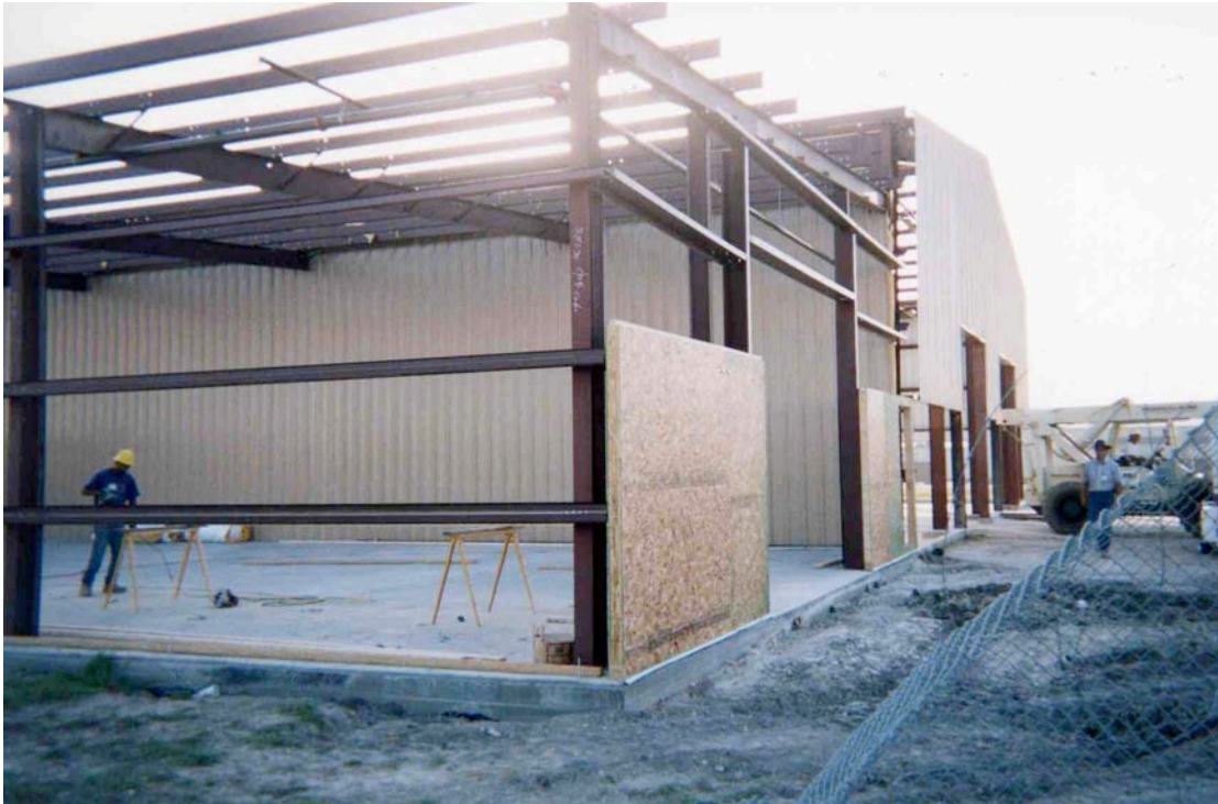
This Agriboard building shows the individual panels of compressed wheat straw and how they're put together.
