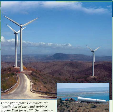
These photographs chronicle the installation of the wind turbines at John Paul Jones Hill, Guantanamo Bay. The four wind turbine towers are about 185 feet high. The blade lengths are 90 feet. The top of the blades are about 275 feet off the ground. The blades rotate at a maximum of 22 RPM, or a rotation every three seconds. This translates to a blade tip speed of 140 mph.
