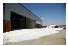
A validation test of the high expansion foam system is performed at the 188th Fighter Wing's new consolidated maintenance facility. It recently received a LEED Silver certification by the U.S. Green Building Council. (U. S. Air Force photo by TSgt. Stephen Hornsey).
