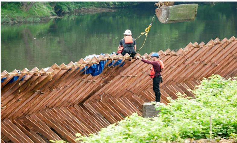
*Site 1 remedial action – cofferdam installation prior to soil removal*
