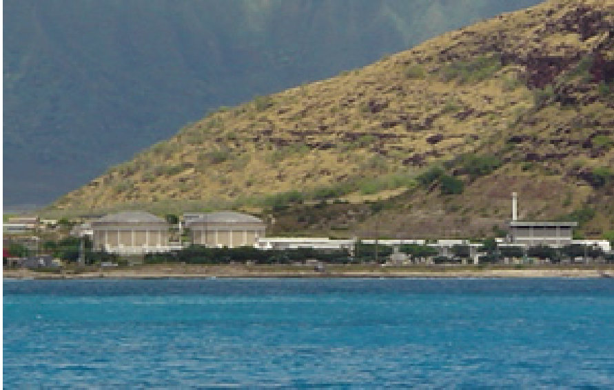
Figure 4. The Wai'anae Wastewater Treatment Plant (WWTP) , Source: CZM Hawai'i
