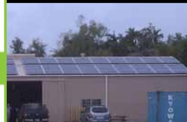
*Before the photovoltaic array was installed at Camp Katuu, PACOM and A/249th Engineering Battalion designed and incorporated modifications to reinforce the roof to support the additional weight of the solar panels and mounting equipment, currently estimated to be 10,500 pounds.*
