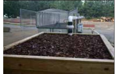
*A biofilter distributes composting discharge air into a manifold and up through pine bark nuggets.*
