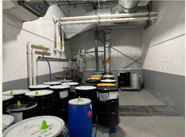
Waste Oil Storage Onsite
