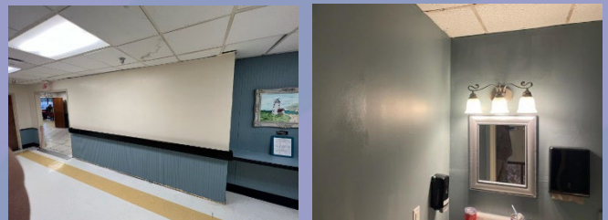
Paint with anti-mold additive demonstrated at Tallahassee Memorial Hospital and Wakulla Springs nursing home (right)
