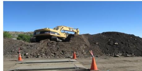
Asbestos-contaminated soil stockpiled for disposal. YPIT 2011.
