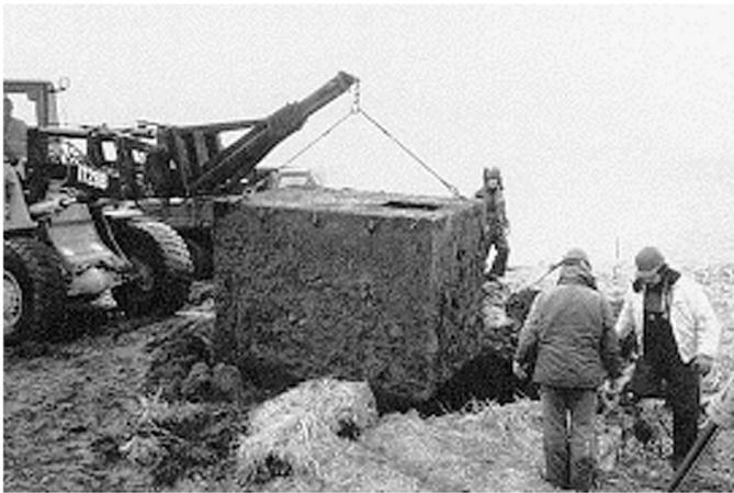
Containerized hazardous, toxic, and radioactive waste (underground storage tank)
