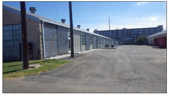
Figure 34. West elevation of building showing the rehabilitated original windows and doors in place. [Note these doors no longer are functional but were left in place to avoid adverse effect to exterior.], 2019 (Texas Military Department).
