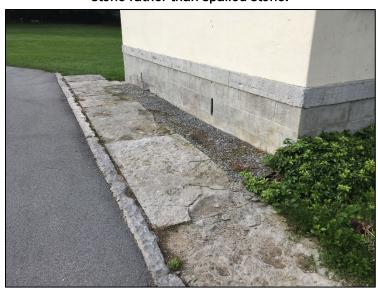
Figure 53. Photograph showing the deteriorating Trenton Limestone pavers (Fort Drum). This material does match our local limestone, but in this form, it is too friable to serve as a walkway. Some of the pavers cracked during installation, others began to deteriorate during the first freeze thaw cycle after installation. Deterioration was exacerbated dramatically by use of de-icing material, but the walkway was too dangerous to be cleared by using only manual snow and ice removal methods.
