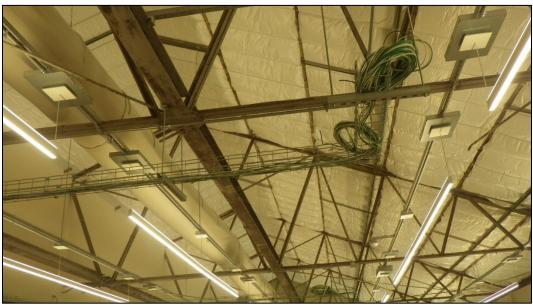
Figure 31. Cable trays for Building 38 were in original design but the connecting posts to bring cables to cubicle drops had to be added when floor outlets were not included in finishing of floors, 2019 (Texas Military Department).
