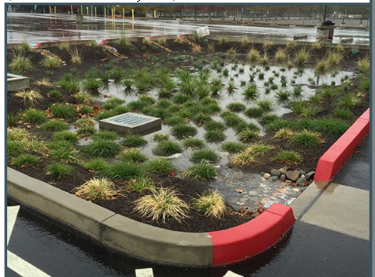
Bioretention planter, Sacramento, CA, 2016 (Source: Sacramento State University)
