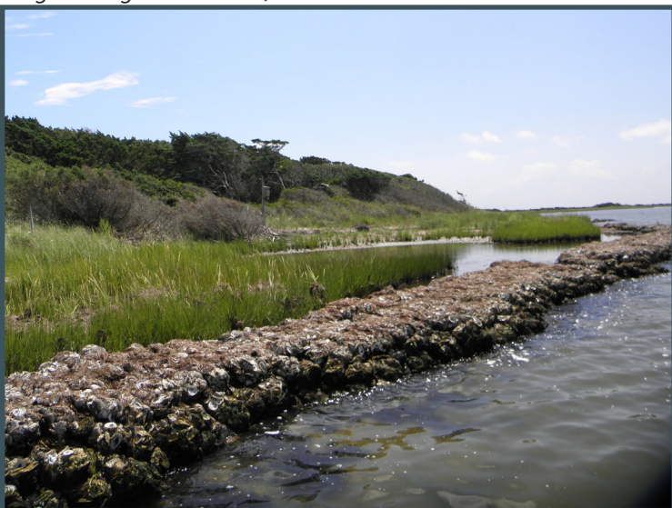
Living shoreline using oyster shells, Ocracoke, NC, 2016 (Source: Ocracoke Observer)
