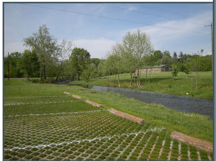
Permeable paver parking lot on greenway, Luray, VA, 2017 (Source: downtownluray.com)
