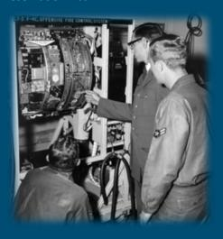
An Instructor at Lowry AFB, Colorado, Explains **Elements of the F-4C Offensive Fire Control System**
