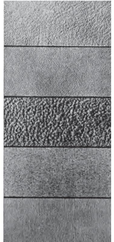
*Illustration 6: Concrete could be finished in various ways. Shown here are examples of hammer finished (top three) and bush-hammered (bottom two). The rougher textures are best adapted to coarse aggregate (Atlas Portland Cement Company 1927:37).*
