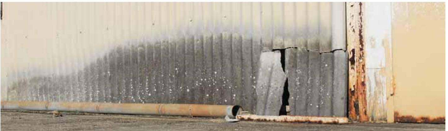
*Illustration 82: Detail of the staining, erosion, discoloration, and lichen growths on Building 448, indicative of degradation (Photographer: Samantha Driscoll 2015).*
