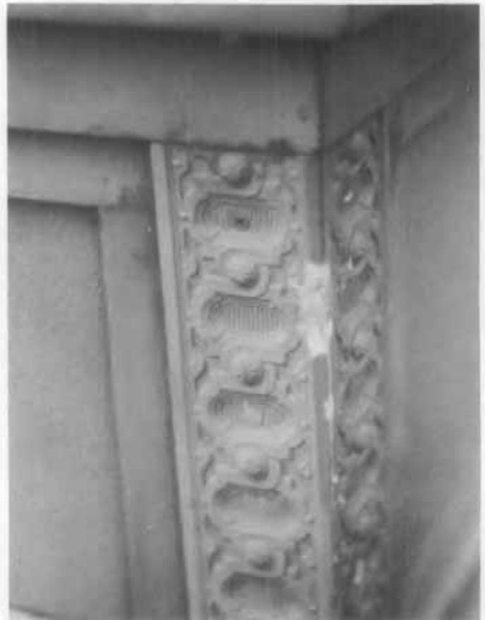
*Illus. 20. Long-term performance can be affected by where the substitute material is located. In this case, fiberglass was used as part of a storefront at street level. Due to the brittle nature of the material and the frequency of impact likely to occur at this location, an unsightly chip has resulted. Photo: Sharon C. Park, AIA.*
