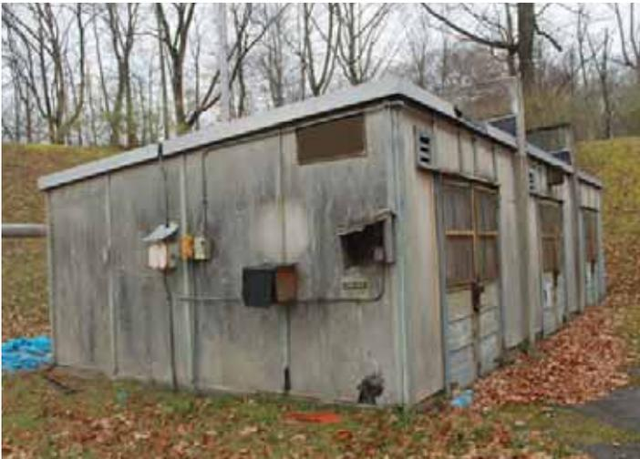
*Illustration 77: Building 1507 at Picatunny Arsenal is clad in flat panel asbestos-cement that is heavily stained, indicating degradation (Photographer: Samantha Driscoll 2015).*
