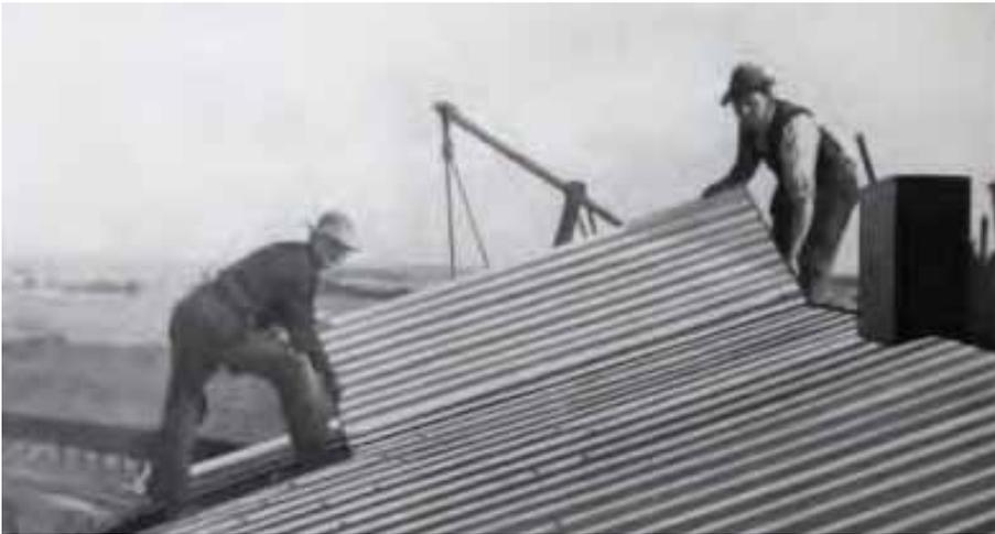
Illustration 30: The application of asbestos-cement corrugated roofing on a steel structure (Kearsby & Mattison Company 1918:28).
