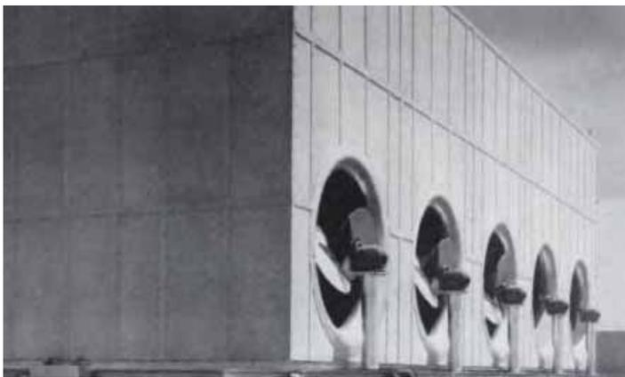
*Illustration 24: An example of flat asbestos-cement panels on a cooling tower (Johns-Manville 1944:13).*
