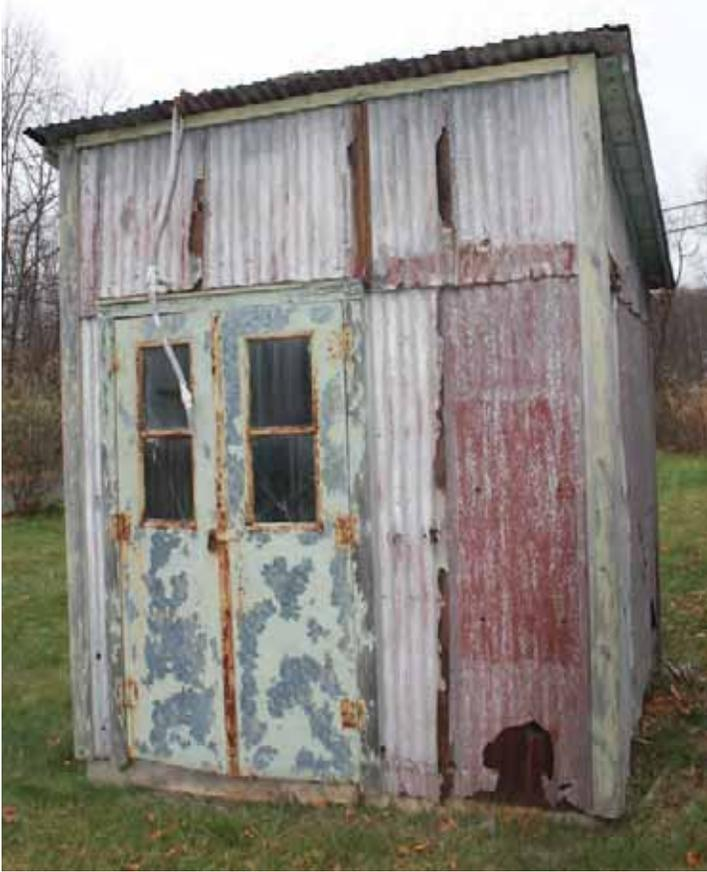
*Illustration 68: Building 1504A at Picatinny Arsenal has suffered a lack of maintenance, resulting in corrosion (Photographer: Samantha Driscoll 2015).*
