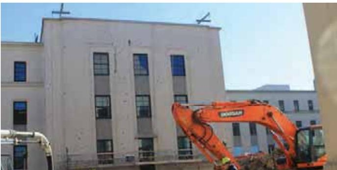
*Illustration 63: Building 3 at NSA Bethesda during repair work to correct cracking, spalling, and exposed reinforcement (Photographer: Samantha Driscoll 2015).*
