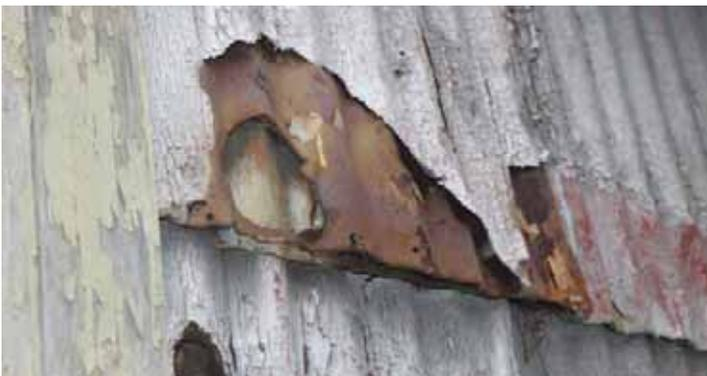
*Illustration 70: Corrosion is not just an aesthetic issue, it can make the material unstable. As seen here, the corrosion has caused a hole in the corrugated steel (Photographer: Samantha Driscoll 2015).*
