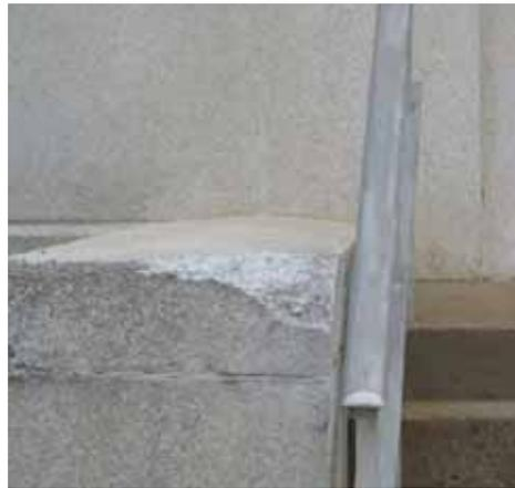
*Illustration 54: An example of spalling on Building 3 at NSFC (Graves 2012).*
