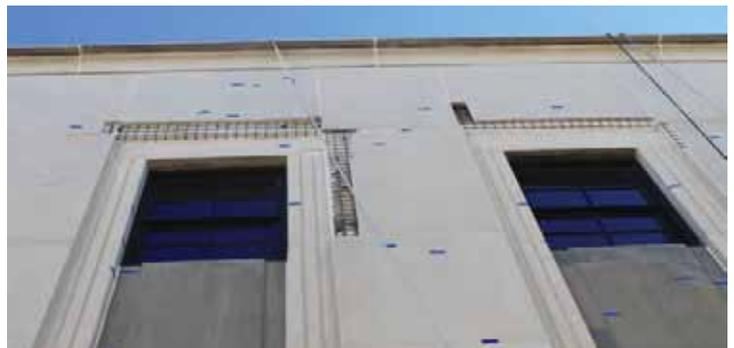
*Illustration 64: Detail of the corroded and exposed steel reinforcement on Building 3, which caused the de-lamination and spalling of the surface concrete. Wire mesh and stainless steel bars will be inserted in these areas prior to patching for stability (Photographer: Samantha Driscoll 2015).*
