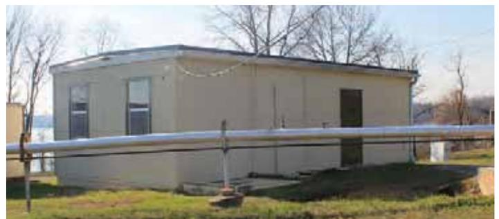
*Illustration 85: Building 544D has flat panel asbestos-cement, which was set to be replaced, but instead was maintained through sealing and painting (Photographer: Samantha Driscoll 2015).*
