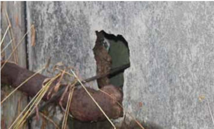
*Illustration 79: Detail of a crumbled section of asbestos-cement located around a corroded pipe on Building 1507 at Picatunny Arsenal, indicating moisture as the cause (Photographer: Samantha Driscoll 2015).*
