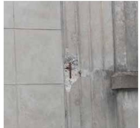
*Illustration 55: Corrosion of steel reinforcement, as shown in this example from Building 173 at Picatinny Arsenal, is a common cause of spalling (Photographer: Samantha Driscoll 2015).*
