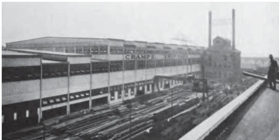
Illustration 27: Asbestos-cement corrugated siding was ideal for large buildings, especially those in harsh environments like this shipyard building in Philadelphia, Pennsylvania (Keasbey & Mattison Company 1918:11).
