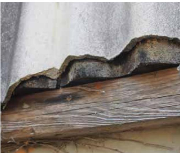
*Illustration 84: Detail of the corrugated asbestos-cement wall where the material has crumbled off. Note the thinness of the asbestos-cement panels, as well as the exposed insulation layer (Photographer: Samantha Driscoll 2015).*
