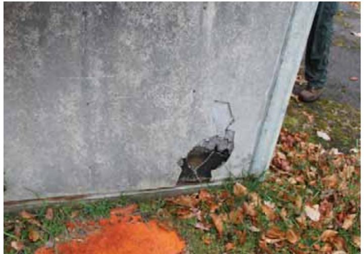
*Illustration 78: Detail of a crumbled section of asbestos-cement on Building 1507 at Picatunny Arsenal (Photographer: Samantha Driscoll 2015).*
