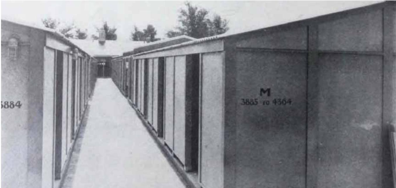
*Illustration 40: Buildings often integrated both flat and corrugated asbestos-cement panels, as seen here (Johns-Manville 1944:28).*
