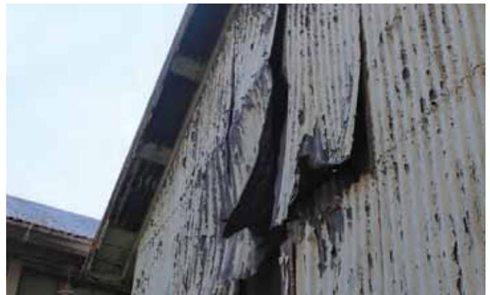
*Illustration 72: Building 179 also has distortion of its corrugated steel cladding, which may have occurred from weather or physical damage (Photographer: Samantha Driscoll 2015).*
