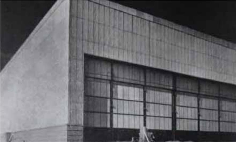
*Illustration 38: An example of a curtain wall constructed with flat asbestos-cement panels (Johns-Manville 1944:32).*
