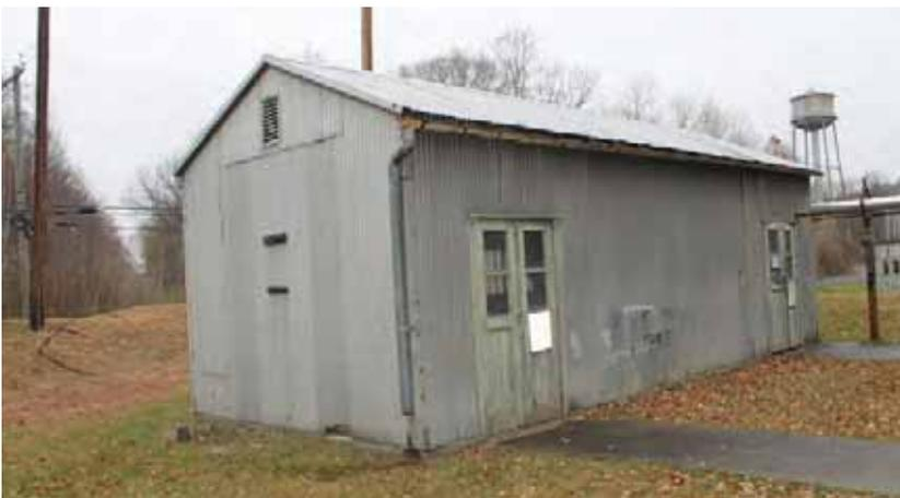
*Illustration 73: Building 1506 at Picatunny Arsenal is clad in corrugated aluminum. In the center of the front elevation is a patch of in-kind material fitted with incompatible fasteners (Photographer: Samantha Driscoll 2015).*
