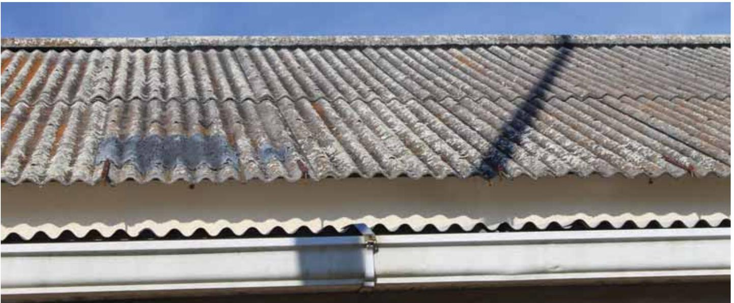
*Illustration 76: Building 466 at NSF Indian Head has a corrugated asbestos-cement roof with degradation. The material has begun to break down and looks rough, which may release asbestos fibers (Photographer: Samantha Driscoll 2015).*
