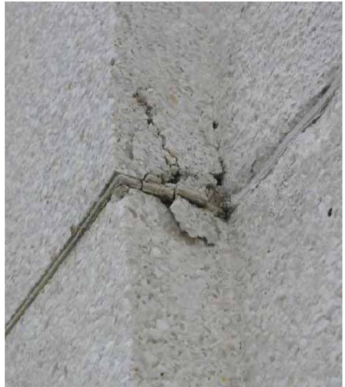
*Illustration 52: An example of a pop-out around a joint on Building 1 at NSFC (Graves 2012).*
