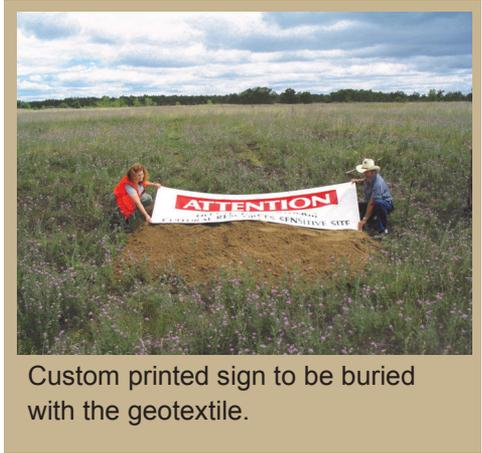
Custom printed sign to be buried with the geotextile.
