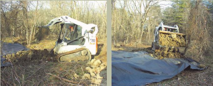
Covering the Horton Store site at USMC Quantico, Virginia, involved covering a majority of the site with geotextile fabric and clean fill. These photographs exhibit the correct way to apply and spread topsoil over fabric.
