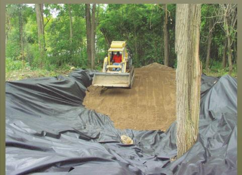
*From top to bottom: Laying geotextile fabric across a site, beginning to place clean sand fill on the fabric, continuing to put clean fill atop the fabric.*
