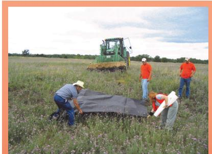
Laying geotextile fabric and clean sand over the geotextile.
