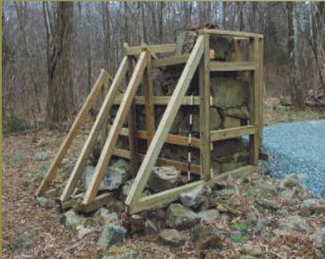
*The Stafford Store at USMC Quantico. From top to bottom: before vegetation removal, cleared foundation during treatment, supported and treated foundation.*
