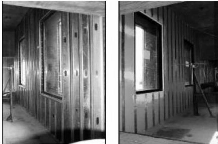
Figure 38. Steel stud partition system (Coltharp and Hall 2002).
