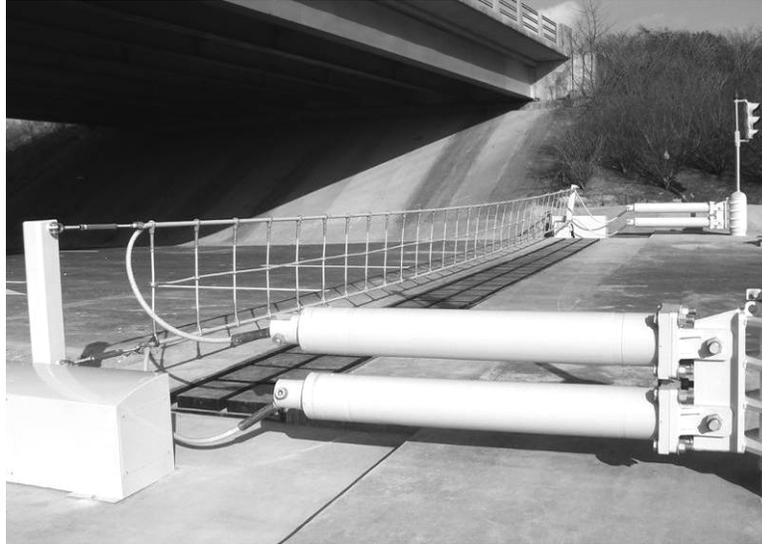
Figure 10. Above-grade components of vehicle net barriers may create a visual challenge when installed in a historic landscape (Universal 2005).
