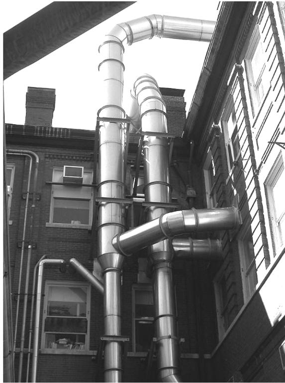
Figure 46. Modern mechanical systems can negatively impact historic properties (ERDC-CERL 2005).
