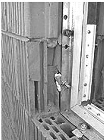
Figure 43. Window anchors in clay tile masonry (ENR 2003).
