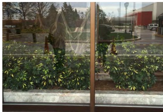
An example of where a potential bird hazard has been created by placing plants inside of a building near the window. Photo by USFWS
