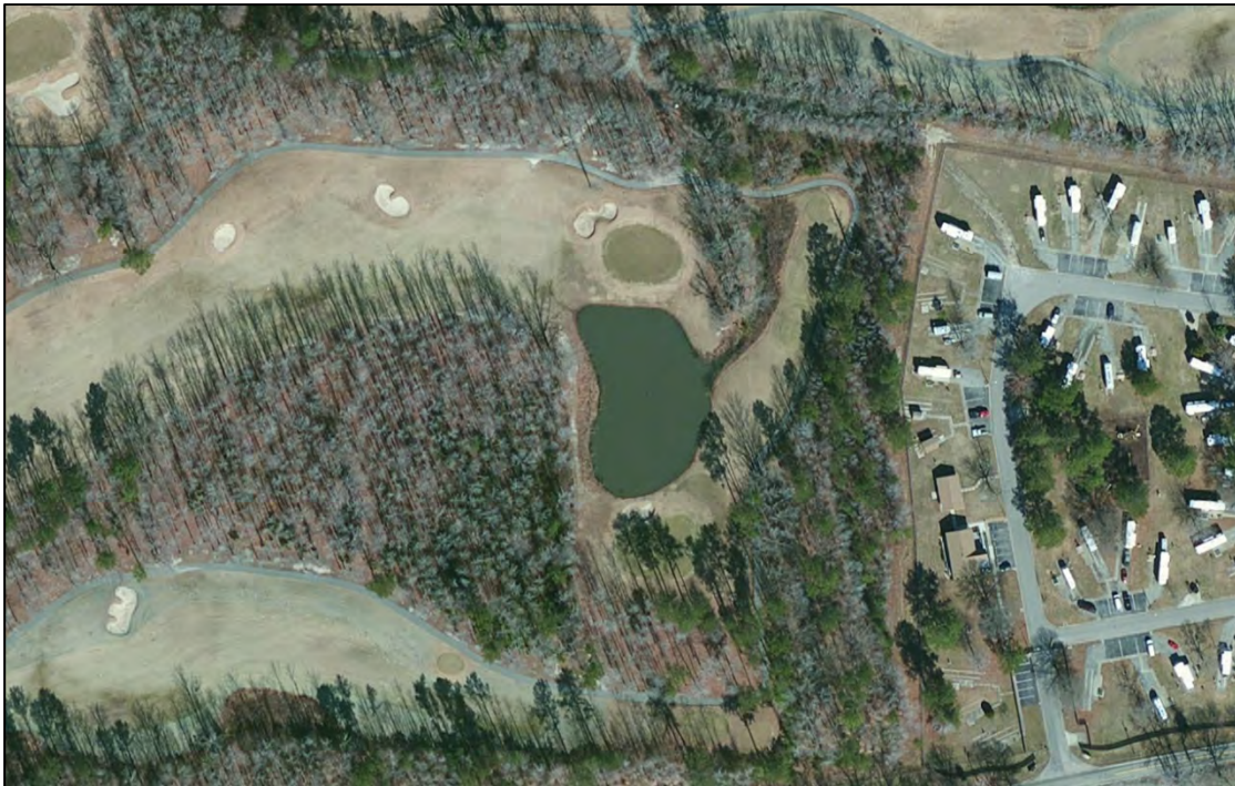
Figure 6. Aeropines Golf Course Pond 3 (Source: Services.arcgisonline.com/arcgis/services/ )
