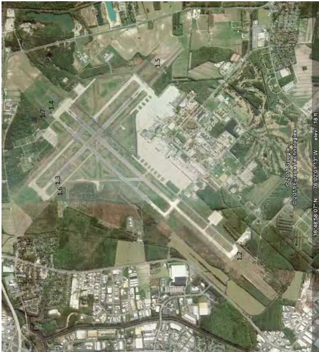
Figure 20: Specific areas on the airfield with poor or improper drainage allowing for extended periods of standing water.
