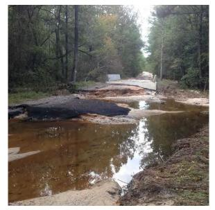
Figure 1: COL Creek Bridge after 2015 Storm (22" of rain in 48 Hours)
