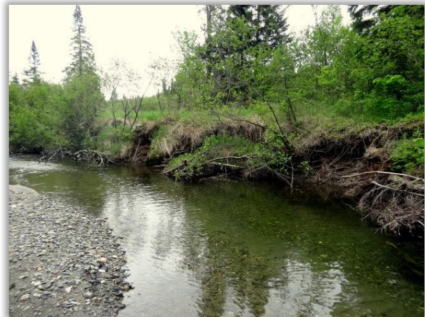
Redington Stream erosion
