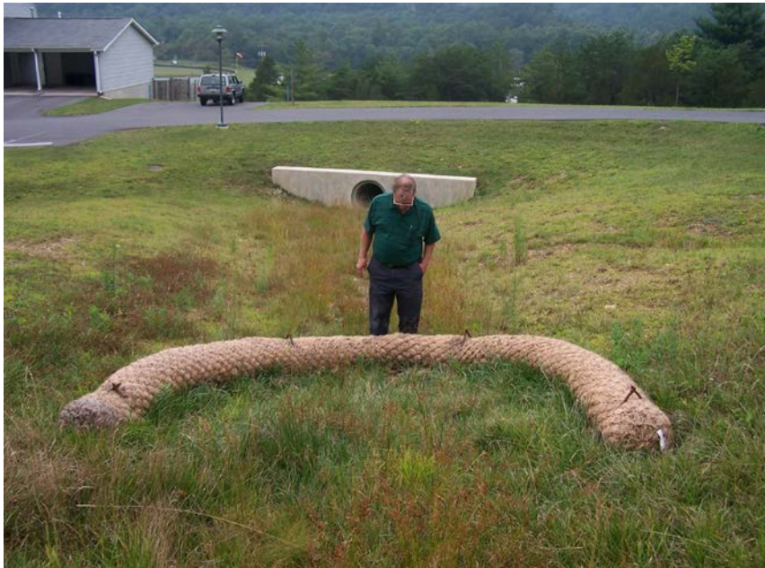
Inspection of biolog installed in base housing area.
