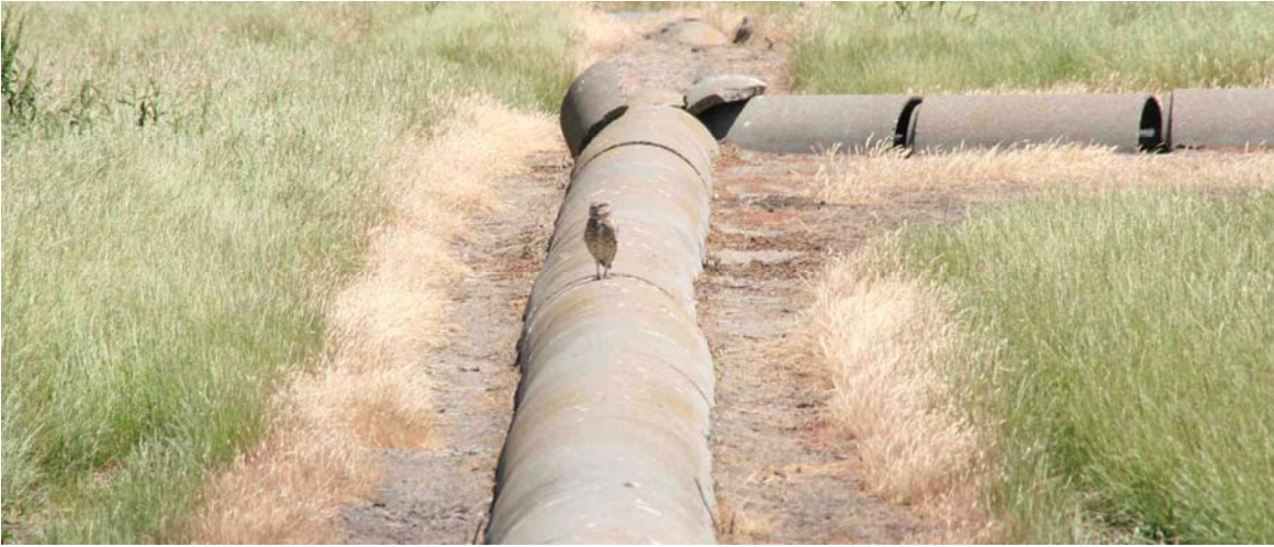
Figure 1. Cable covers are used as nest sites where gaps in the covers allow burrowing owls access to the interior.
