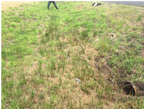
Wetland 4, with drainage culvert to Wetland 5
