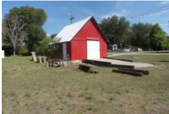
Photograph 2-14. Barn at Southern End of LEFAC/Bugg Spring Facility
