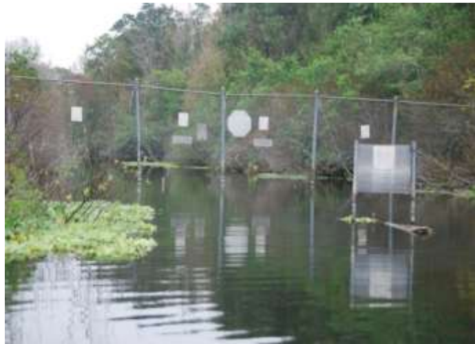
Photograph 2-6. Security Fence Crossing Spring-run Stream Channel
