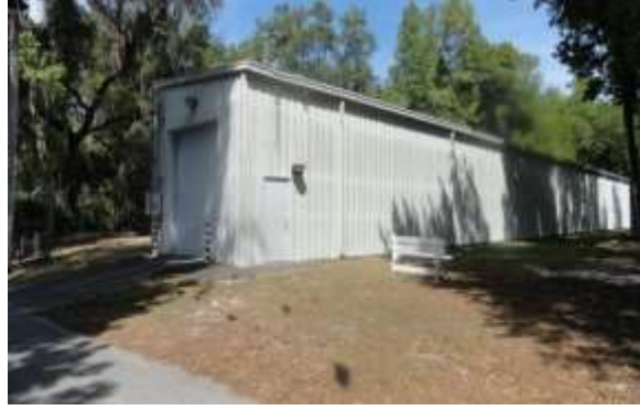
Photograph 2-8. LEFAC/Bugg Spring Storage Building
