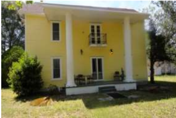
Photograph 2-13. NRHP-Listed House on LEFAC/Bugg Spring Facility
