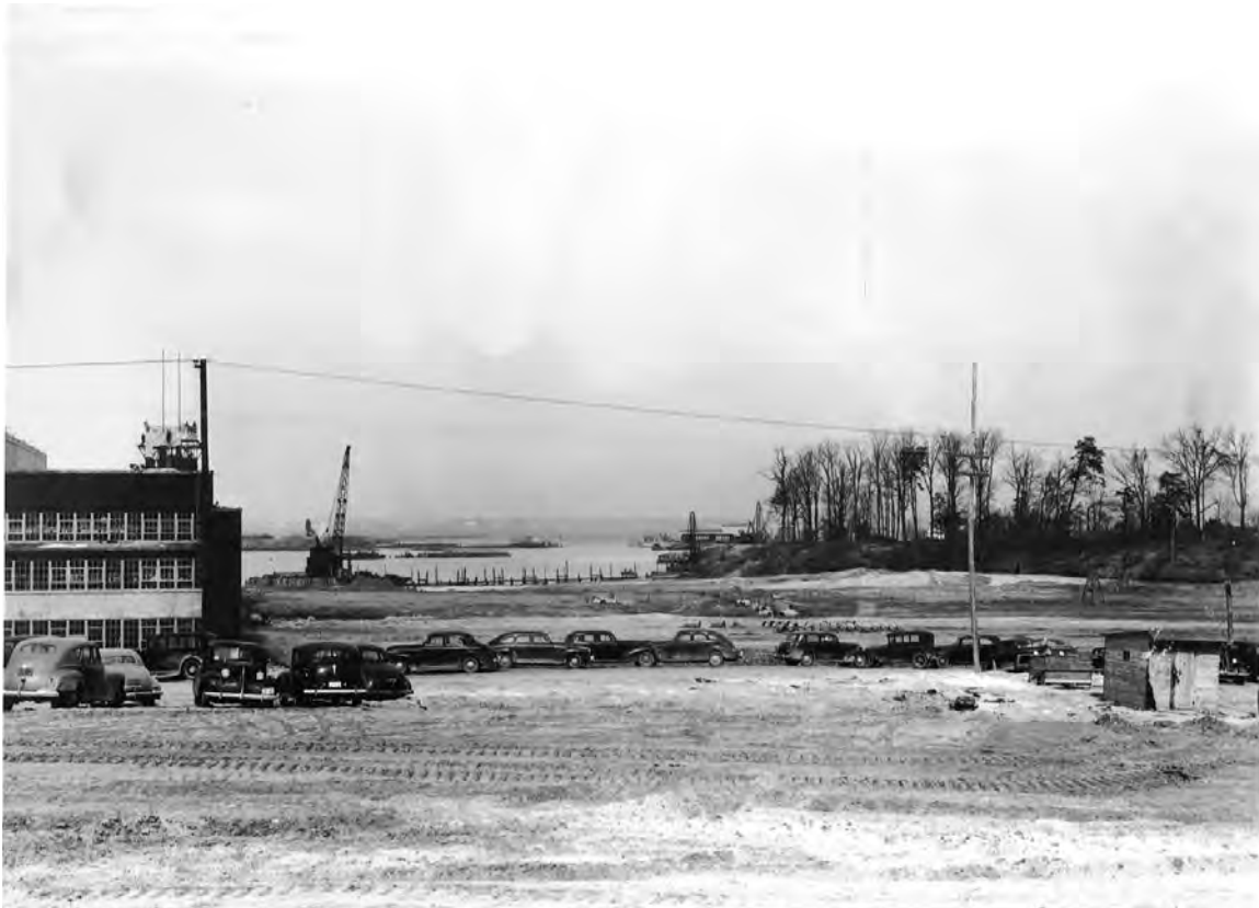
Naval Air Station, Patuxent River, MD. Seaplane Hangar (Steel), Trans. Area. (Project No. 4). View Looking north showing apron. Contractor Cummins Constr. Corp. and Riggs-Distler and Co. Contract NOy-5363. Date 3-1-1943 (PW# 1199)
