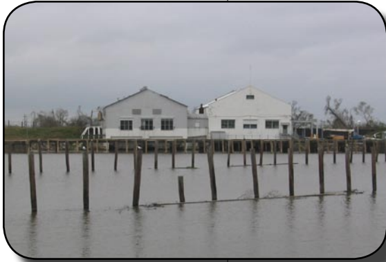
Pumping Station on the Intracoastal Canal
