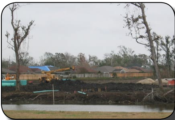
Clearing of Land Near the Back Gate
