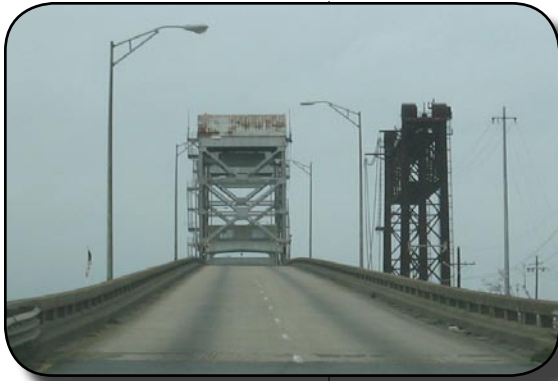
Existing Intracoastal Canal Crossing at LA23
