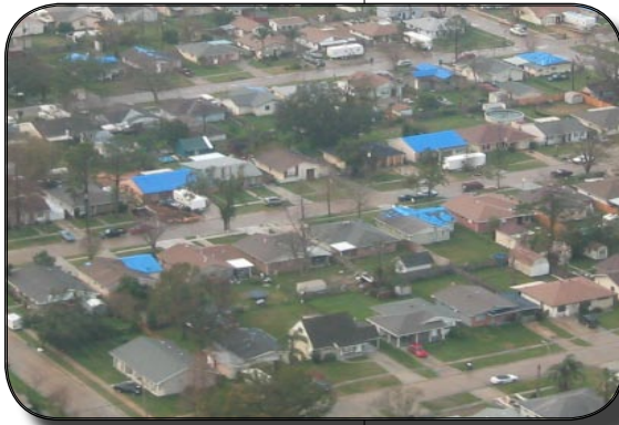
Hurricane Damage to Residential Structures
