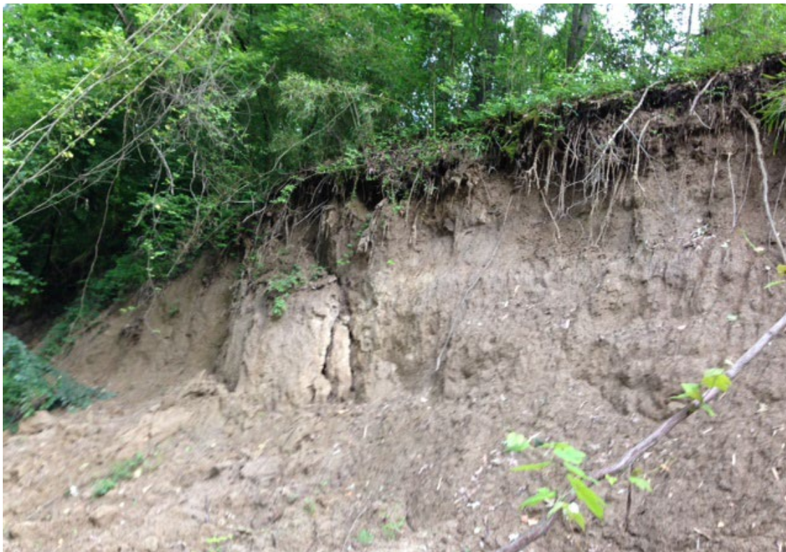
Photograph 6-2. Erosion of along the banks of the Southwest Channel
