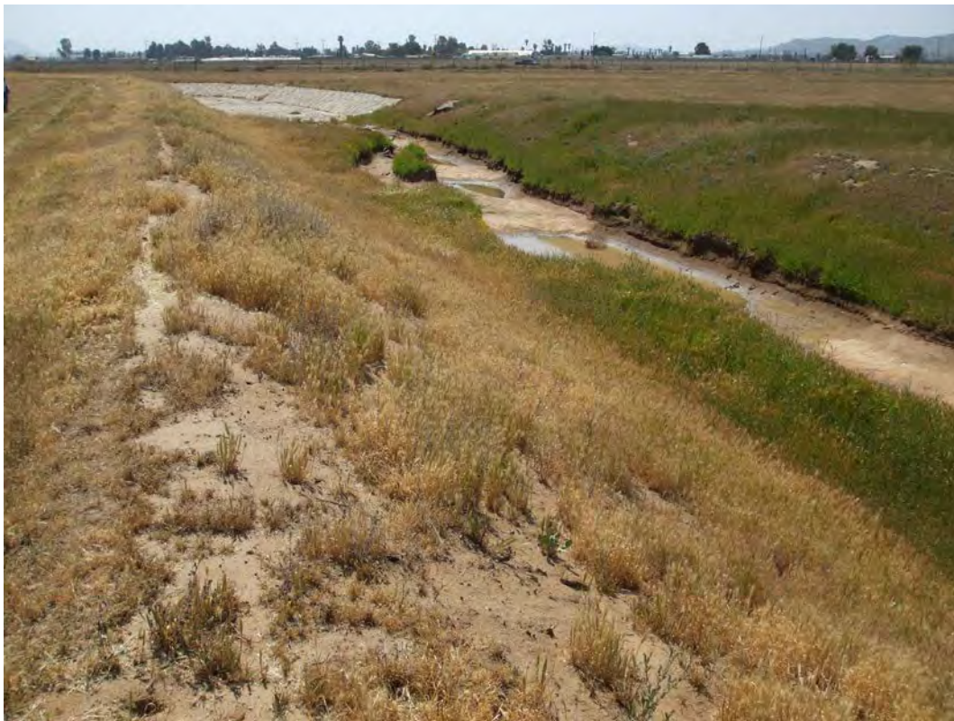
Photo 10 (April 2009): The main drainage that flows through Survey Area 13 at the southern end of March ARB connects with the Harley Knox Boulevard Channel and discharges into the Perris Valley Storm Drain. At this location, the channel changed from dirt with defined bed and banks to a concrete-lined channel.
