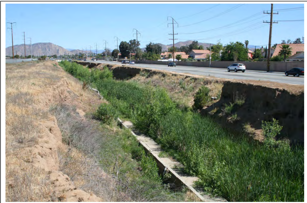
Photograph 3: View looking north, between Cactus Avenue and Meyer Drive. The photo depicts emergent wetland vegetation within Heacock Channel.
