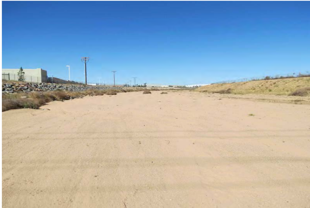
Photograph 2: Photograph depicting the Perris Valley Storm Drain.
