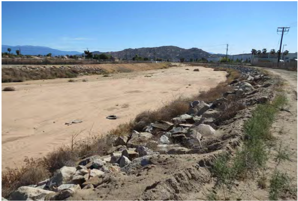
Photograph 1: Photograph depicting the Perris Valley Storm Drain.
