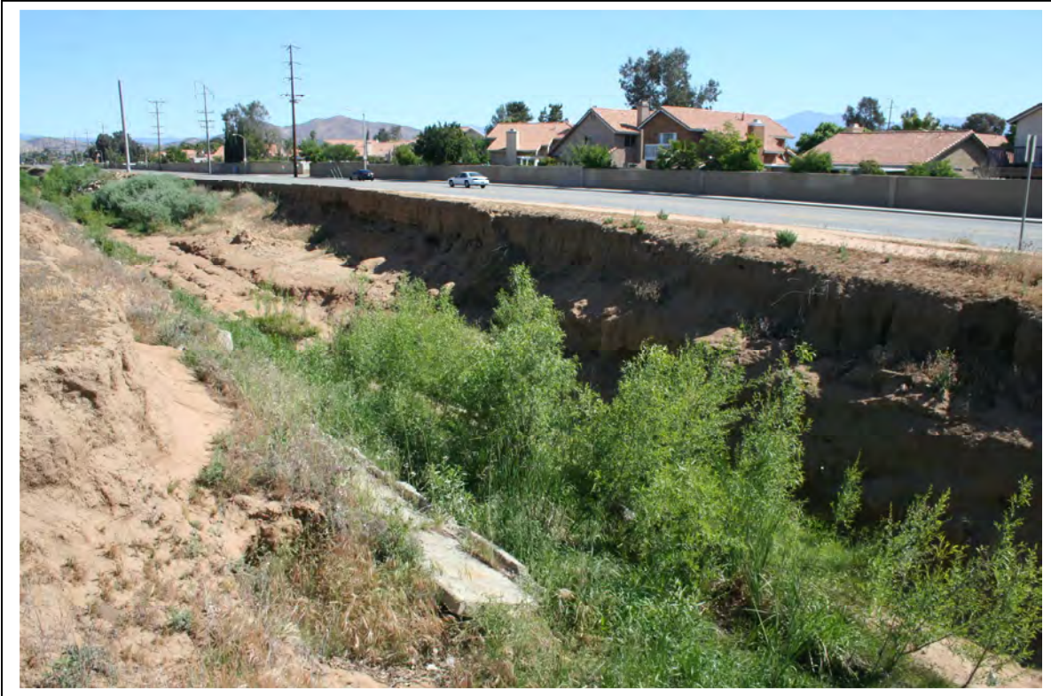
Photograph 1: View looking north, just south of Cactus Avenue. Photo depicts southern willow scrub riparian habitat within Heacock Channel.
