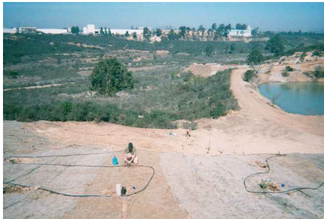
Slope Restoration - Fish Pond Natural Resources Division
