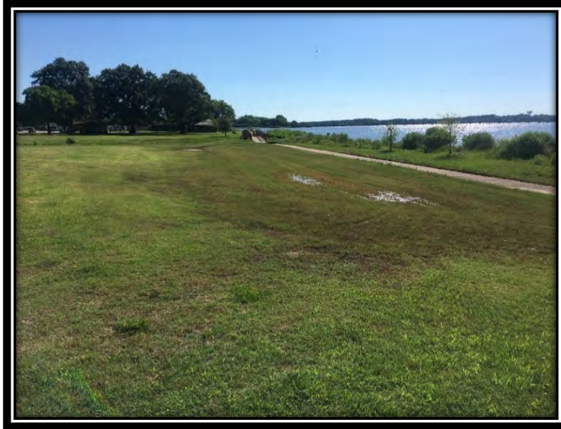
JBLE-Langley Areas Regularly Flooded by Storms and Tides
