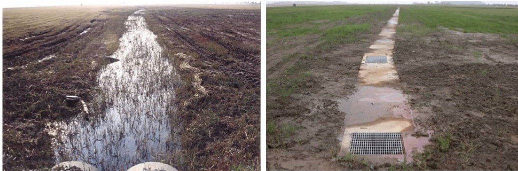
Figure 7.3 Airfield drainage ditch prior to enclosure (left) and above-grade lateral drainage after enclosure.
