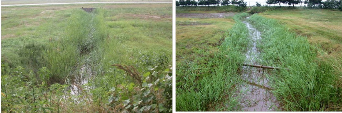
Figure 7.2 Overgrown vegetation impedes water flow (left) and overgrown vegetation creates bird habitat.
