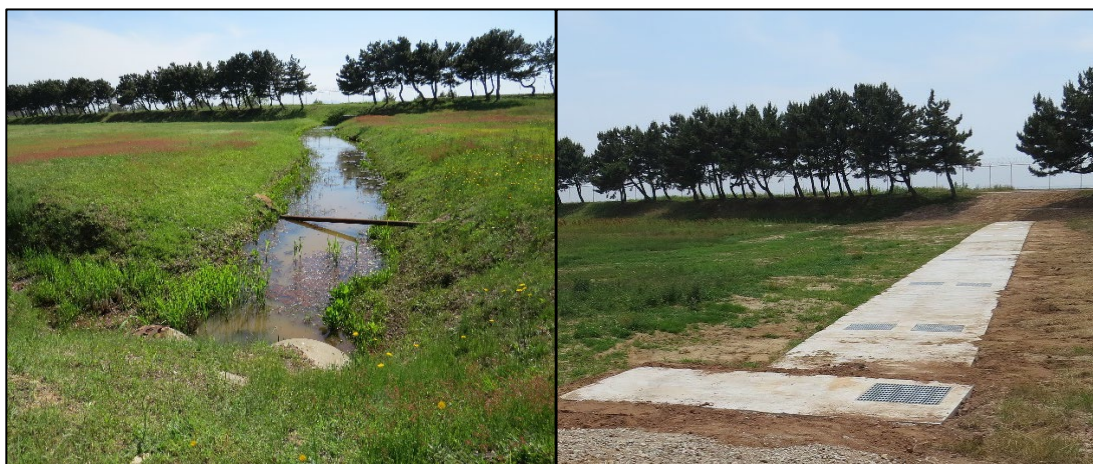
Figure 2.64 Seoul Frog Habitat, Runway Drainage Ditch, 2017 (left) and 2018 (right)
