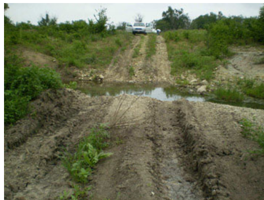
Figure 7: Stream crossing approach damaged by maneuver traffic.
