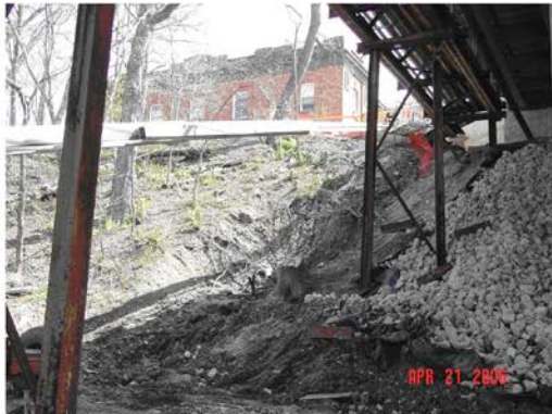
Figure 4-2 Erosion Around Utilities
