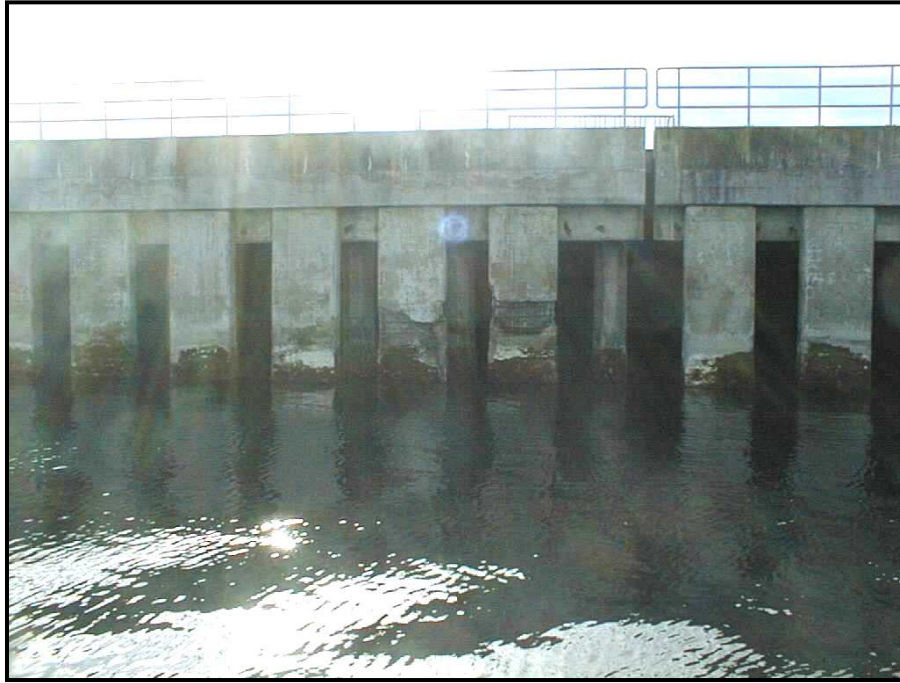
Figure 2-24. Pier B Wave Attenuation Baffles (Source: NAVFAC)
