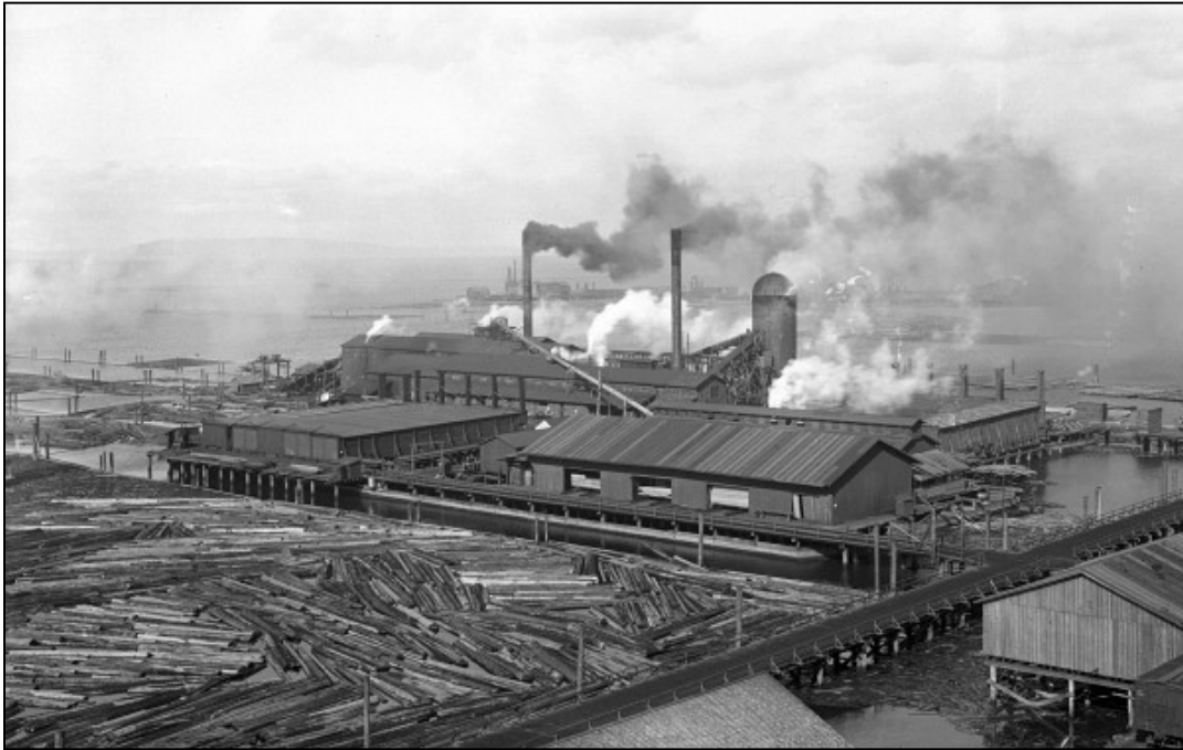
Figure 2-4. Clough-Hartley Mill, 18th Street, ca. 1915 (Source: Everett Public Library)
