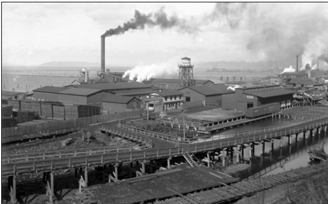
Figure 2-5. Robinson Manufacturing, 21st Street, ca. 1915 (Source: Everett Public Library)
