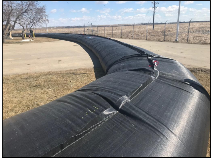
Figure 4-1. AquaDam deployed at NRTF LaMoure to provide temporary control of flooding.
