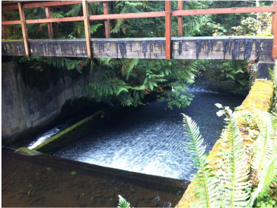
Figure 11. Cub Creek dam, forming Cub Creek reservoir.
