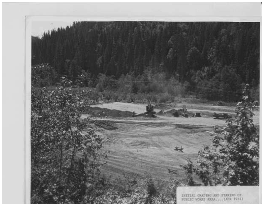
Figure 2. Initial grading for public works area, approximately 1951.
