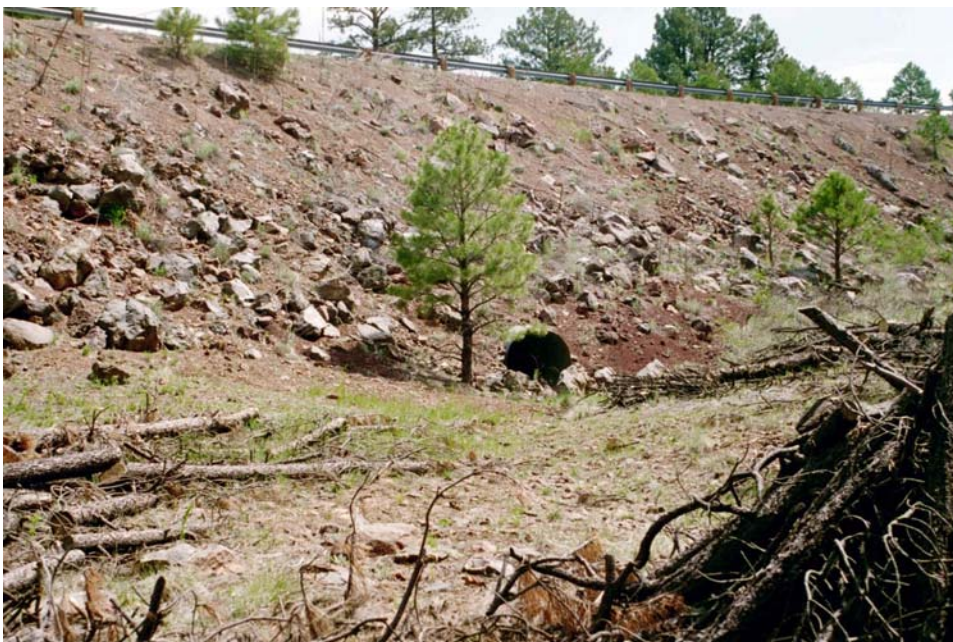
Photo 13. Area 2, road culvert, Waters of U.S. Check 1, jurisdictional.
