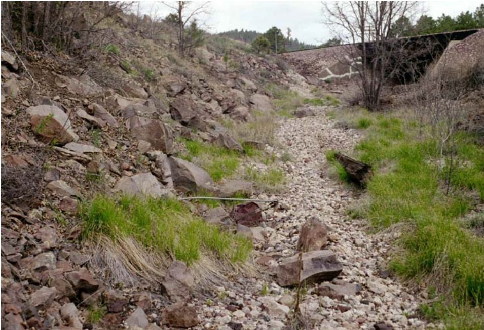
Photo 8. Area 1, drainage under railroad track.
