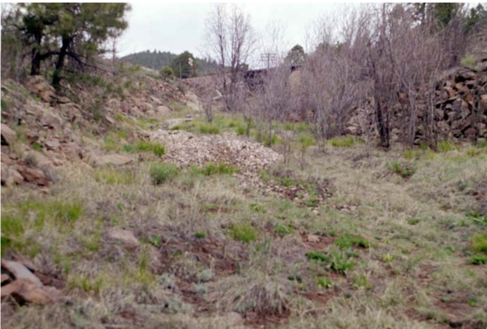
Photo 3. Site 1, railroad drainage.
