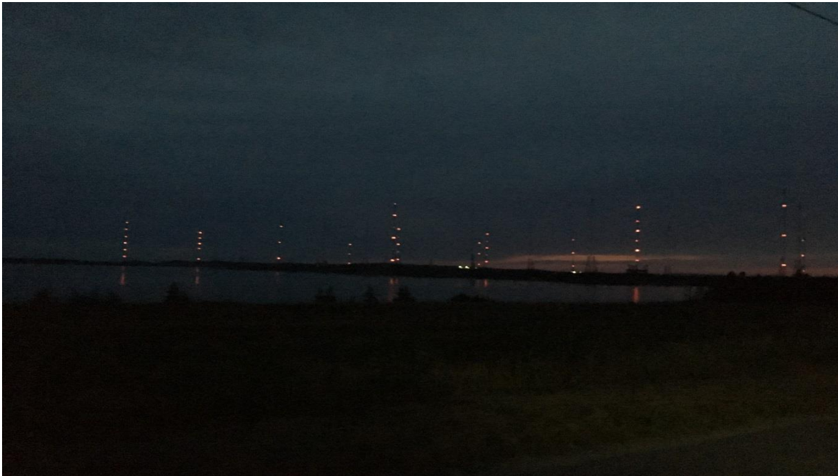
Figure 4. Image of the Installation at Nighttime, NCTAMSLANT DET Cutler.
