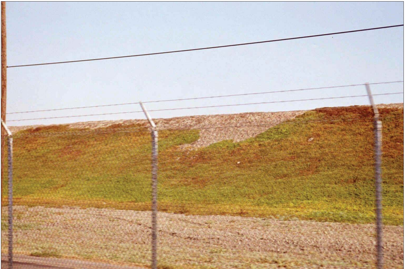
Photo 2-6. Magazine slope, showing planted iceplant, which has been considered for all magazines as a means to control erosion.
