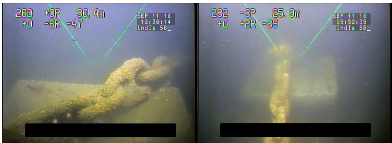
Figure 11. Still images taken from ROV survey video showing the FSB anchor blocks and chains.
