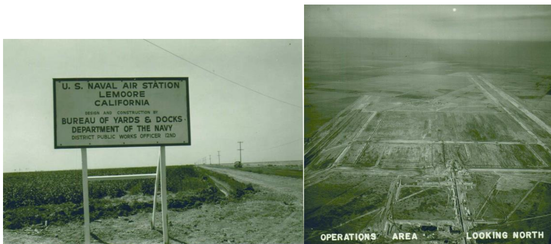
Photo 2-1. Naval Air Station Lemoore Main Gate during Station construction in 1958 (Left). Looking north at the Naval Air Station Lemoore Operations Area while under construction in January 1959 (Right).
