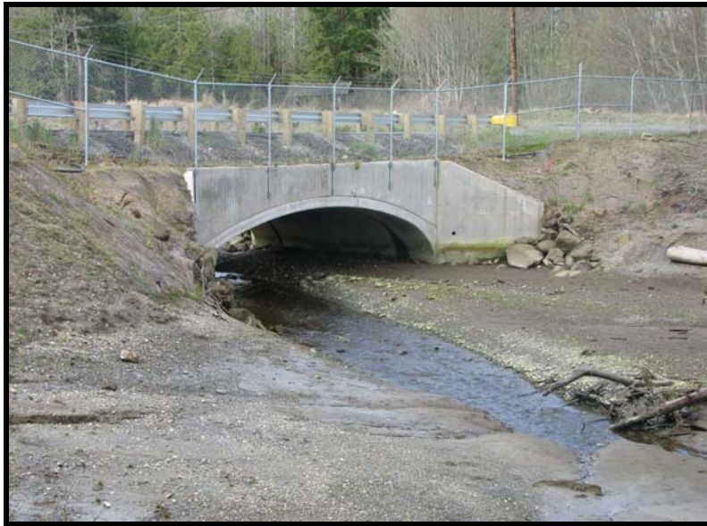
Figure 2-6. New Arched Culvert at the Mouth of Beaver Creek.
