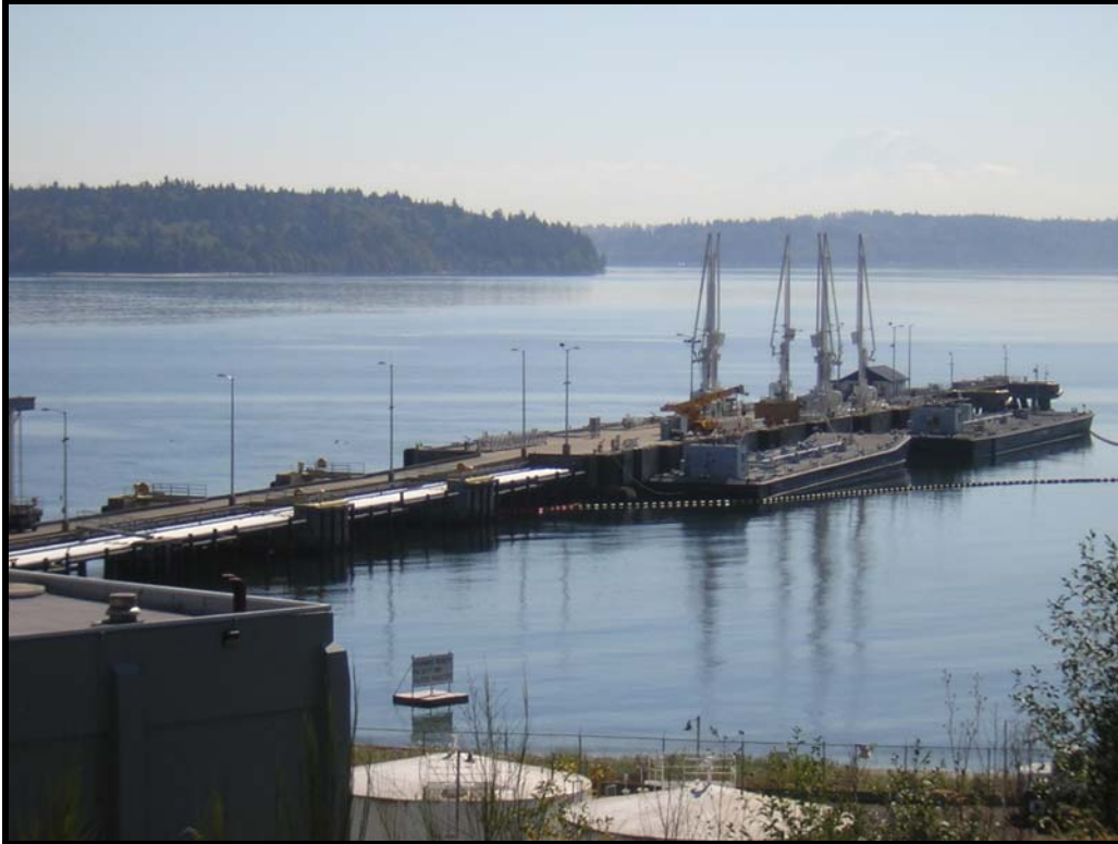
Figure 2-1. Manchester Fuel Department – Fuel Pier.
