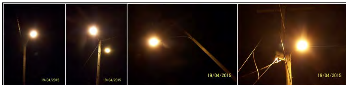
Figure 7. Examples of gold-peach light, indicative of high-pressure sodium lamps identified at Joint Expeditionary Base Fort Story
