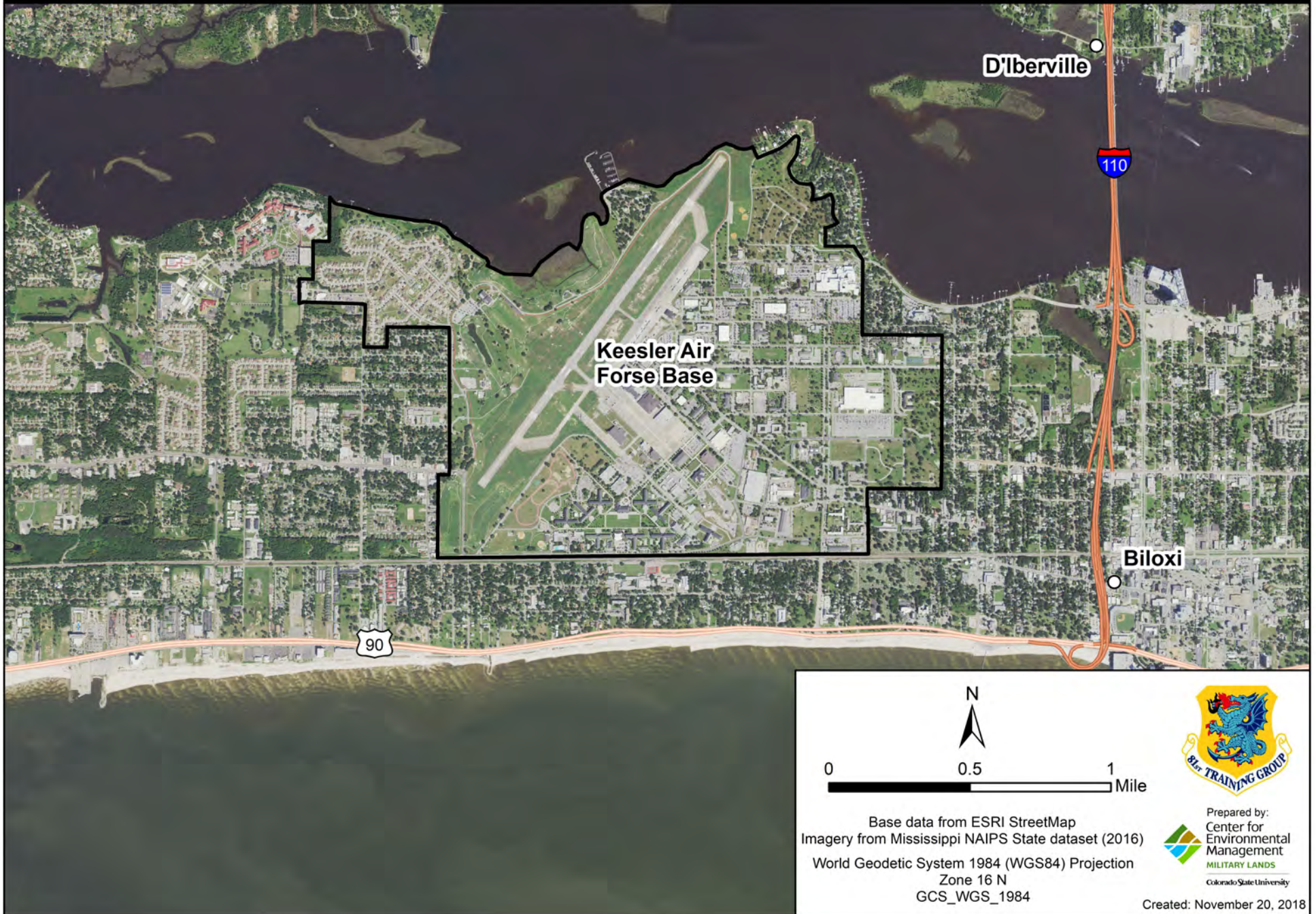
Figure 2-2. Aerial image of Keesler Air Force Base
