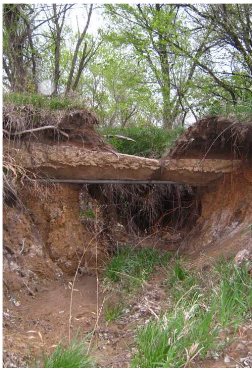
Figure 13: Uncovered Utilities at MAFB Figure 14: Bank sloughing along a mowed stream.
