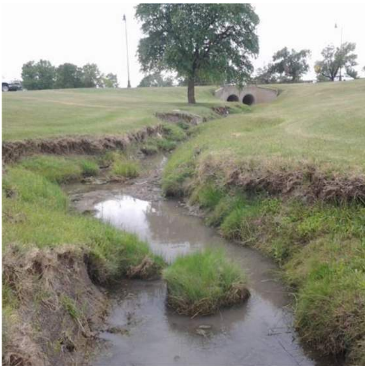
Figure 13: Uncovered Utilities at MAFB Figure 14: Bank sloughing along a mowed stream.
