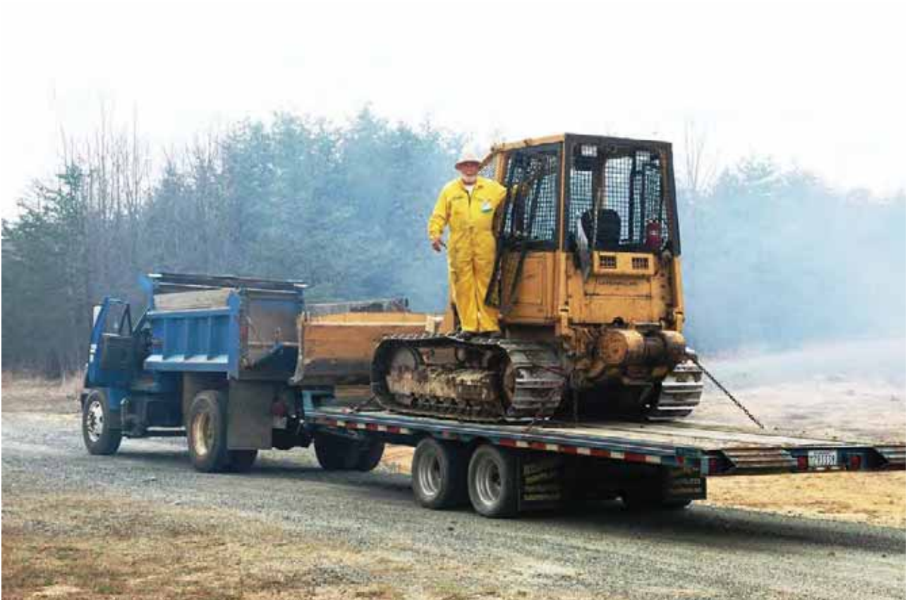
Small bulldozer standing by on a prescribed burn, which could be utilized to establish a firebreak and help with spot fires that often occur.
