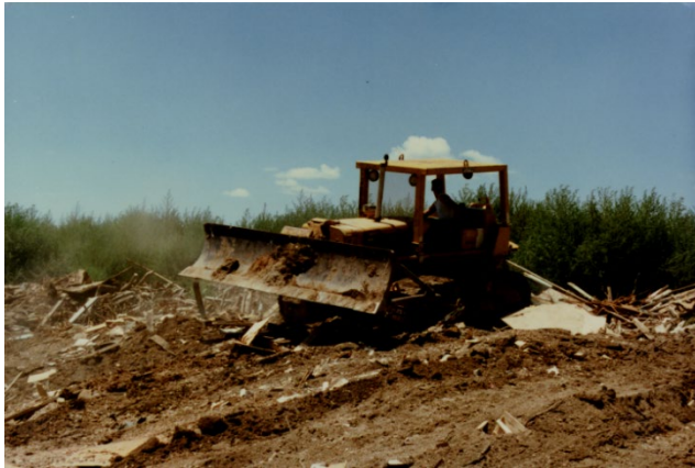
Covering of Materials- South Landfill.
