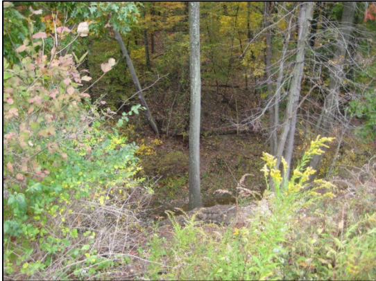
Area 5 – Location of outfalls and bad erosion.
