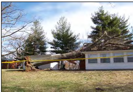
Figure 15. Failed Oak Tree in Cole Park.
