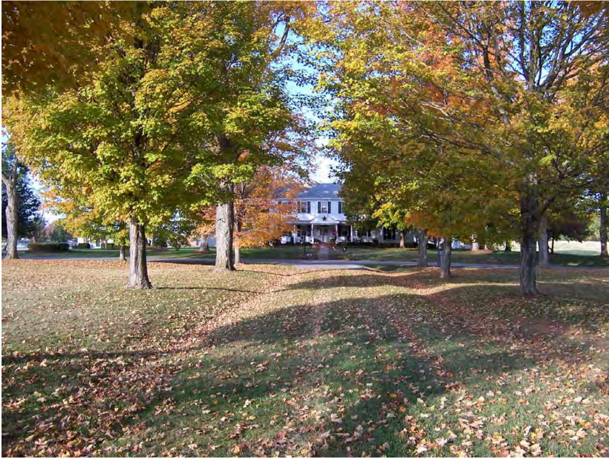
Figure 6. Commanding General's Residence
