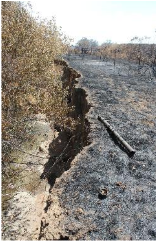
Photo 18. Streambank erosion, Fallbrook Creek, 2014. (Photo by C.M. Wolf)
