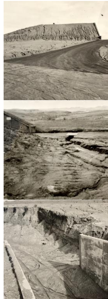
Photo 10. Archive photos of excessive magazine erosion due, in part, to lack of vegetation, circa 1950s-60s.
